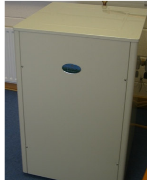
Water-to-Water (Well) Geothermal Heat Pump
